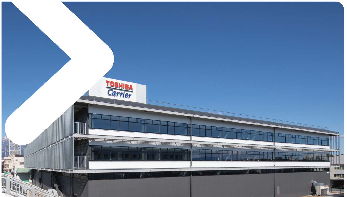
Japan - Fuji Operations R&D Centre e-THIRD building
